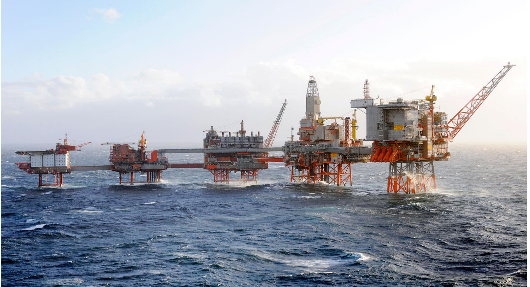
Valhall platform - AkerBP
